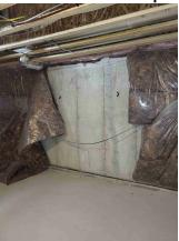
178301 - 3 - 20240826\_145934 - foundation repair that was completed in basement by draintite. wrap required to be replaced - need new blanket wrap - approx 60 feet. - please deliver and instal as my guys dont have the proper equipment to instal this. as per my serviceman, will need a ran set nailer and 3 rolls of tape. see photos
