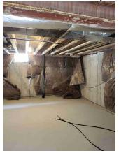
178301 - 2 - 20240826\_145923 - foundation repair that was completed in basement by draintite. wrap required to be replaced - need new blanket wrap - approx 60 feet. - please deliver and instal as my guys dont have the proper equipment to instal this. as per my serviceman, will need a ran set nailer and 3 rolls of tape. see photos
