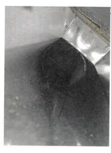
177907 - 3 - 20240623\_173716 - Inspect venting duct in bedroom not connected- No air flow Cut drywall open to expose for National to install new pipe and 90.
