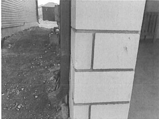
174139 - 1 - NOTE:~CHIPPED BRICK LEFT OF LEFT GARAGE DOOR AT CORNER
