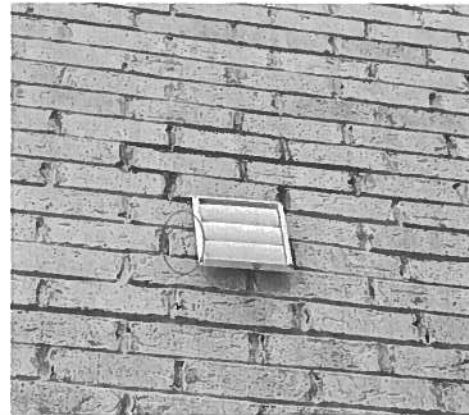
176627 - 1 - Item #57 - crack on 1 brick next to a kitchen vent on a left house side
