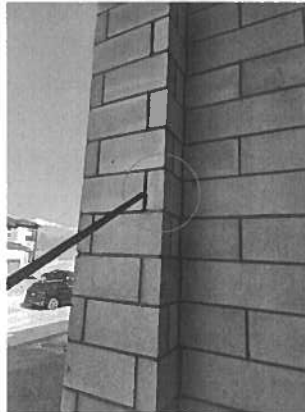
176576 - 1 - #6 - rough stone cut inside the porch on the left- side at stairs
