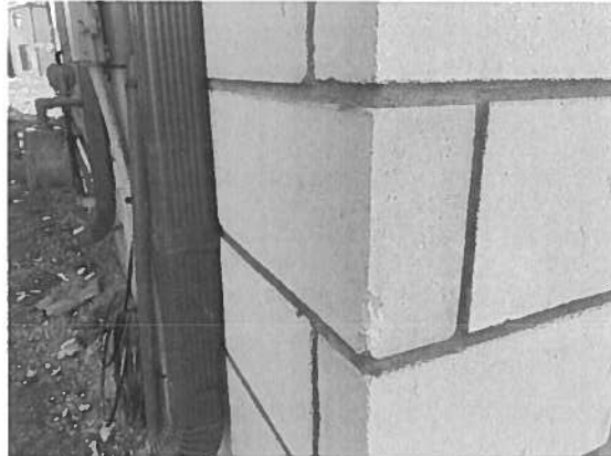
174139 - 2 - NOTE:~CHIPPED BRICK LEFT OF LEFT GARAGE DOOR AT CORNER
