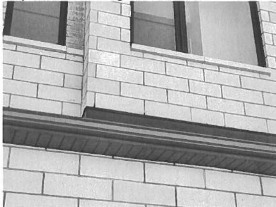
176574 - 1 - ITEM #4 - under front window stone chip-above flashing
