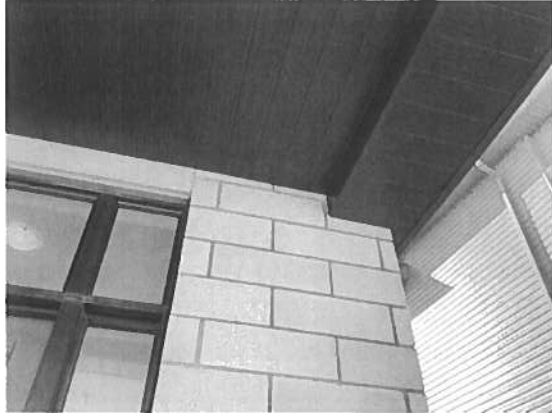
174125 - 2 - NOTE:~CHIPPED BRICK AT RIGHT COLUMN RIGHT OF FRONT DOOR AT SOFFIT
