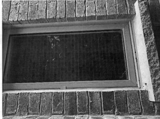
162371 - 2 - IMG_1585 - remove mortar from windows throughout
