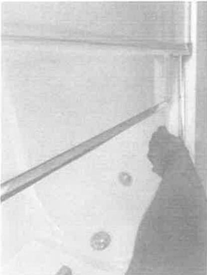
162100 - 1 - TUB~REMOVE YELLOW STAIN FROM INSIDE TUB.
