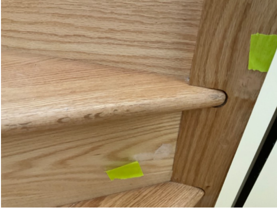
170973 - 1 - STAIRS~VARNISH REQUIRED AT 3RD RISER FROM MAIN FLOOR
