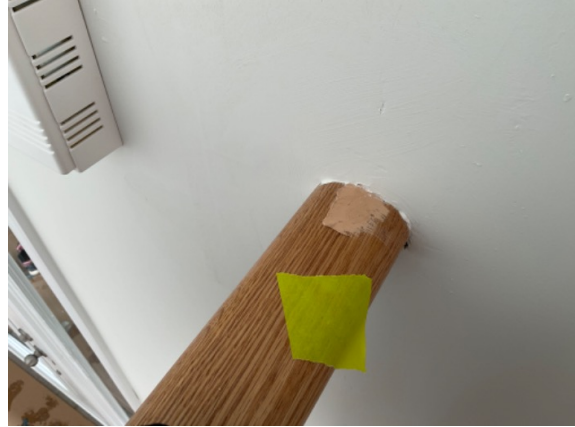
170974 - 1 - STAIRS~SAND AND TOUCH UP VARNISH AT HAND RAIL
