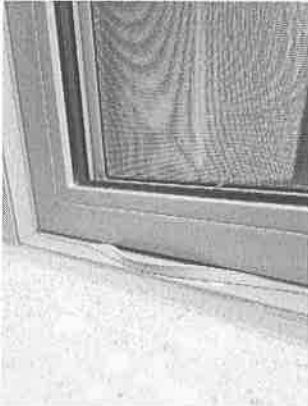
169027 - 1 - ITEM 6 - EXTERIOR GLASS/WINDOWS \\ Exterior trim Condition: Living room window seal is ripped/loose at bottom of operable window. Location: Living Room As per item 7 of Home Inspection report
