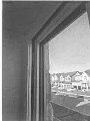
169080 - 1 - item #49 - Right side operable window is warped. Location: Bedroom 3 As per item 54 of home inspection report
