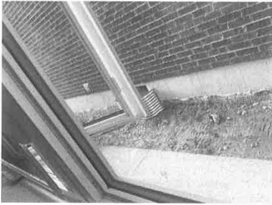
164548 - 1 - WINDOWS~RUBBER SEAL ON WINDOWS LOOSE
