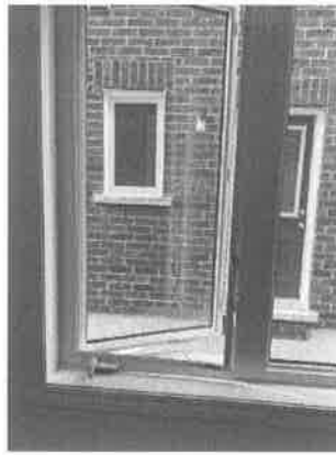
164548 - 2 - WINDOWS~RUBBER SEAL ON WINDOWS LOOSE
