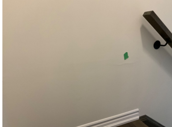
169166 - 1 - WALLS~SEAMS VIABLE AT 1ST LANDING FROM MAIN FLOOR TO 2ND FLOOR
