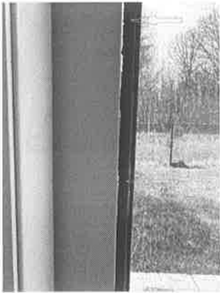
169352 - 1 - Glass 1 - Sliding glass inserts coming out of frame
