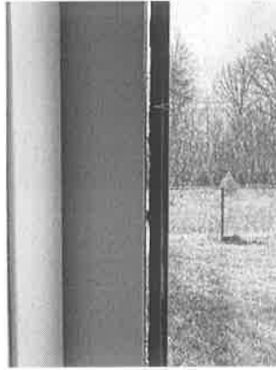
169352 - 2 - Glass 2 - Sliding glass inserts coming out of frame
