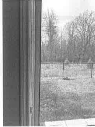
169352 - 4 - Glass 4 - Sliding glass inserts coming out of frame
