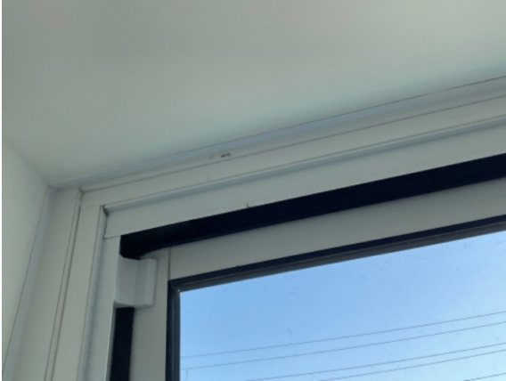
161964 - 3 - NOTE:~DAMAGED MULIN AT SLIDING DOOR AT FIXED GLASS
