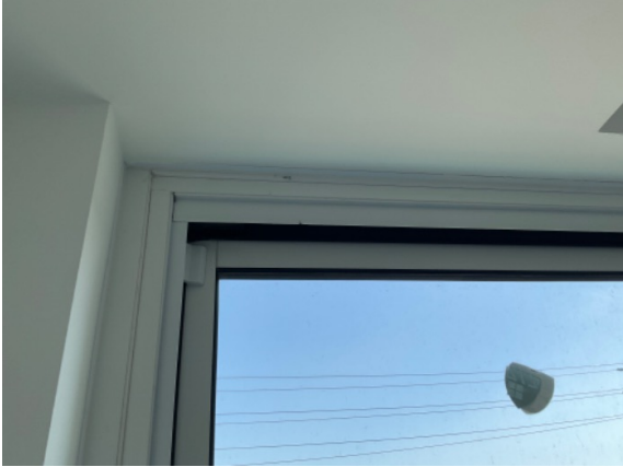
161964 - 1 - NOTE:~DAMAGED MULIN AT SLIDING DOOR AT FIXED GLASS
