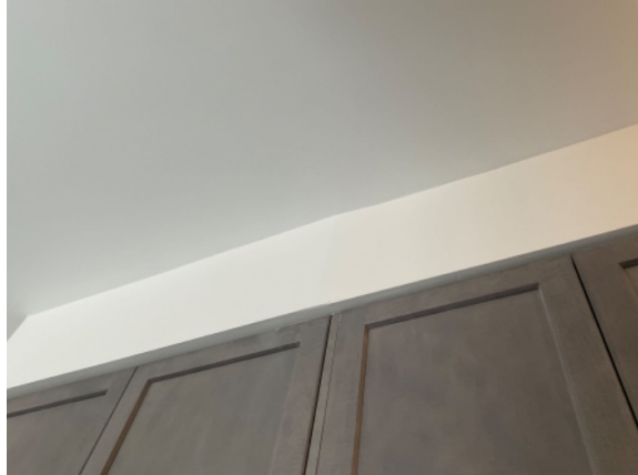
160134 - 1 - CABINETS~SEEM/BULGE AT BULKHEAD ABOVE FRIDGE
