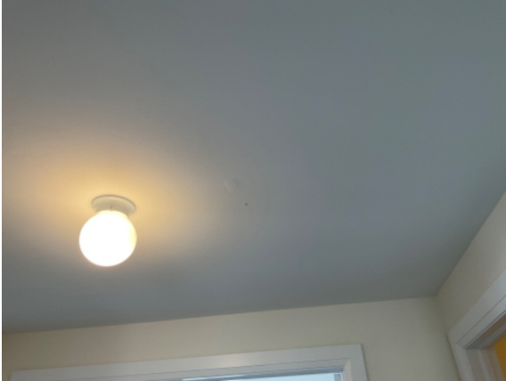
160115 - 1 - WALLS~BULGE IN CEILING INFRONT OF MASTER.
