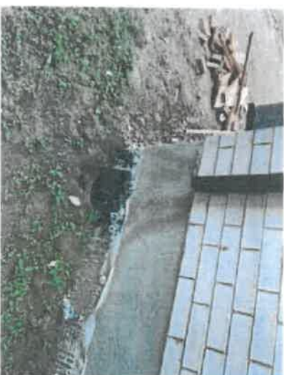
159775 - 1 - NOTE:--ELBOW NOT INSTALLED LEFT SIDE OF HOME
