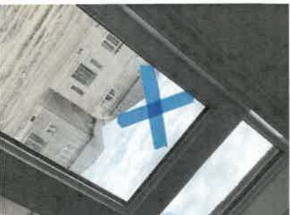
160976 - 2 - WINDOWS~CRACK AT LEFT FIX GLASS ABOVE SINK
