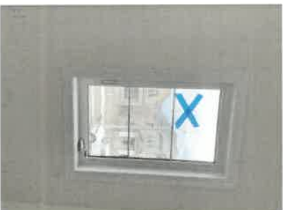
160983 - 1 - WINDOWS~CRACKED GLASS RIGHT OPERATING WINDOW
