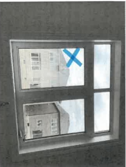
160976 - 1 - WINDOWS~CRACK AT LEFT FIX GLASS ABOVE SINK
