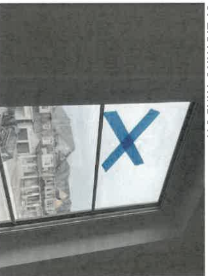
160983 - 2 - WINDOWS~CRACKED GLASS RIGHT OPERATING WINDOW
