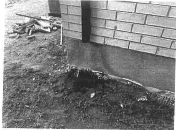
159775 - 1 - NOTE:~ELBOW NOT INSTALLED LEFT SIDE OF HOME
