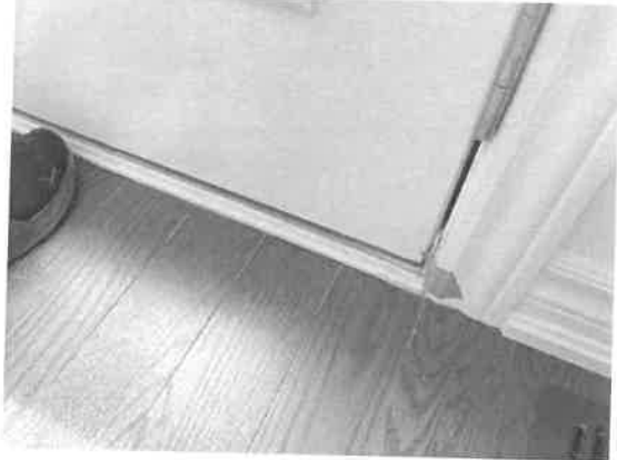
160368 - 1 - TRIM~WATER DAMAGE AT TRIM BELOW BALCONY DOOR.
