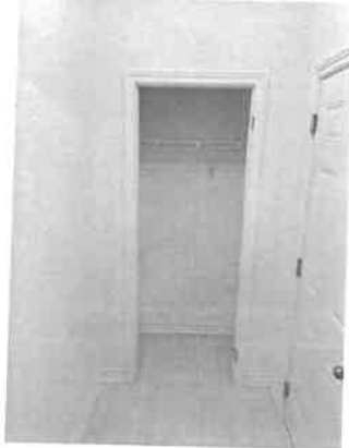
160391 - 1 - CLOSET~DOOR NOT INSTALLED A CLOSET IN MUDROOM
