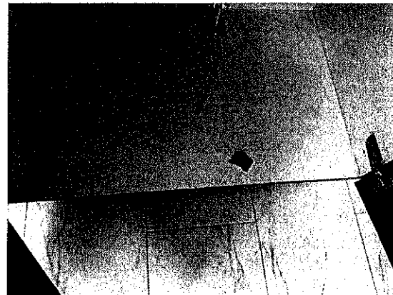
160363 - 2 - VANITY CABINETS~CHIPS ON LEFT AND RIGHT GABLES BELOW SINK
