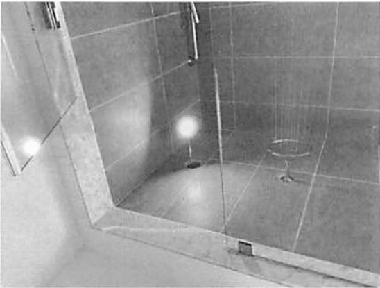
159995 - 1 - ELECTRICAL/LIGHTING~SECURE POT LIGHT INSIDE SHOWER
