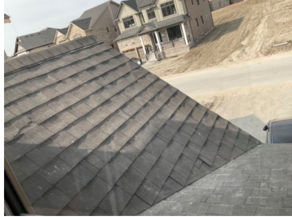
157141 - 2 - SHINGLES~TORN SHINGLES AT ROOF PEAK ABOVE GARAGE CAN SEE FROM BEDROOM 4
