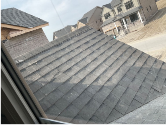
157141 - 1 - SHINGLES~TORN SHINGLES AT ROOF PEAK ABOVE GARAGE CAN SEE FROM BEDROOM 4
