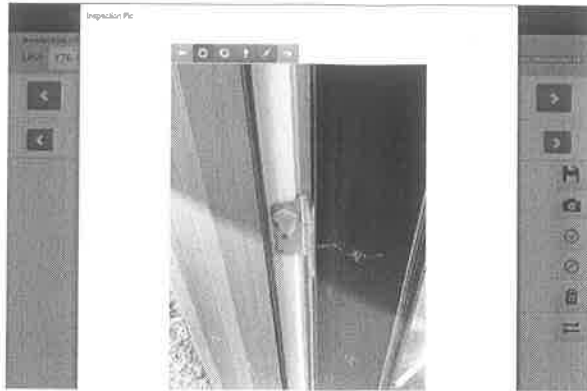
155731 - 1 - IMG_1884 - SCREWS MISSING AT HINGES AT FRONT DOOR
