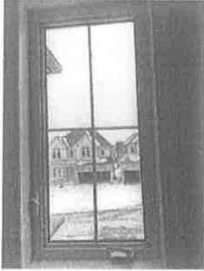
154885 - 1 - WINDOWS~SCREEN NOT INSTALLED AT LEFT WINDOW
