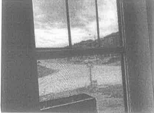
152084 - 1 - WINDOWS~RIGHT OPERATING WINDOW ADJUST FILLER PIECE NOT STRAIGHT
