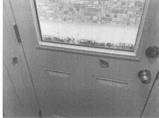
154723 - 2 - NOTE:~DENT ON MAN DOOR BELOW GLASS INSERT
