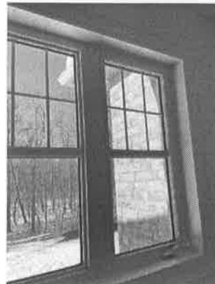
154399 - 1 - NOTE:~INSPECT SCREEN AT OPERATING WINDOW FOR BOW
