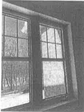
154399 - 1 - NOTE:~INSPECT SCREEN AT OPERATING WINDOW FOR BOW
