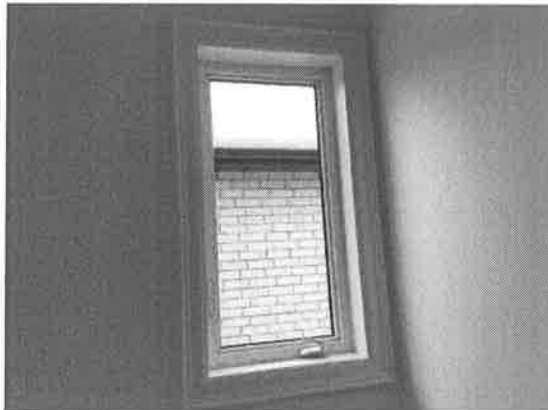
154277 - 1 - WINDOWS~SCREEN NOT INSTALLED AT WINDOW
