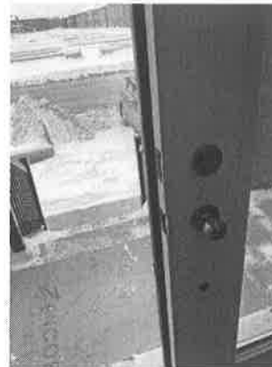
154272 - 2 - FRONT DOORS~REPLACED WEATHER STRIP AT FRONT DOOR TORN 2) OPERATING FRONT DOOR WEATHERSTRIP TO BE REPLACED AT BASE PEELING
