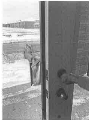
154271 - 1 - FRONT DOORS~CHIPS ON ASTRICAL AT FRONT DOOR
