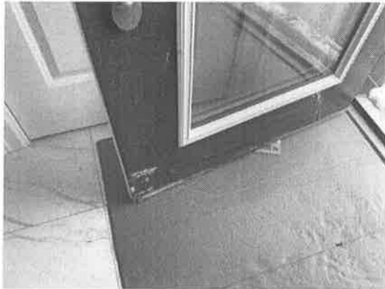
154272 - 1 - FRONT DOORS~REPLACED WEATHER STRIP AT FRONT DOOR TORN 2) OPERATING FRONT DOOR WEATHERSTRIP TO BE REPLACED AT BASE PEELING
