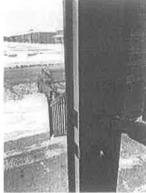
154271 - 1 - FRONT DOORS~CHIPS ON ASTRICAL AT FRONT DOOR
