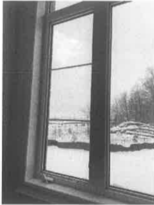
154265 - 1 - WINDOWS~SCREEN NOT INSTALLED AT WINDOW
