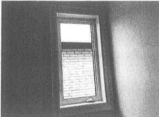
154277 - 1 - WINDOWS~SCREEN NOT INSTALLED AT WINDOW
