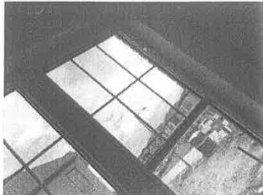
152108 - 2 - WINDOWS~LEFT FIXED WINDOW INSERT FALLING AND INSPECT RIGHT OPERATING WINDOW FOR BEING BOWED
