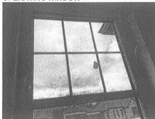
152142 - 1 - NOTE:~SCREEN RIPPED AT OPERATING WINDOW
