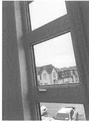
154086 - 2 - WALLS~WINDOW SCREEN NOT INSTALLED AT OPERATING WINDOW
