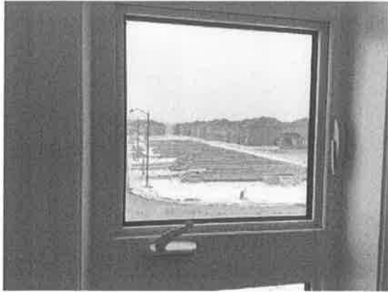
154086 - 1 - WALLS~WINDOW SCREEN NOT INSTALLED AT OPERATING WINDOW
