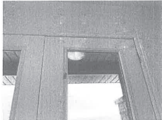
150247 - 3 - FRONT DOORS~SCREW CAPS NOT INSTALLED LEFT DOOR X3
