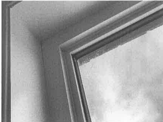
152307 - 1 - WINDOWS~SMALL CHIP AT UPPER LEFT CORNER FIXED WINDOW
