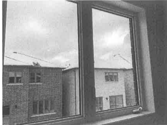
152312 - 1 - WALLS~SCREEN ON WINDOW NOT INSTALLED
