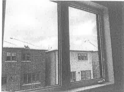
152312 - 1 - WALLS~SCREEN ON WINDOW NOT INSTALLED
