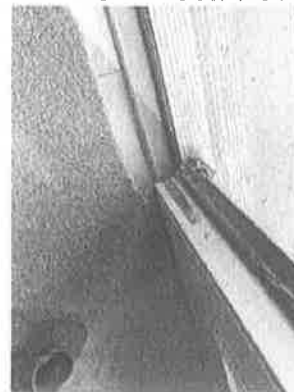
151399 - 1 - FRONT DOORS~FIXED DOOR LOCK NOT WORKING AT BOTTOM OF FRONT DOOR
