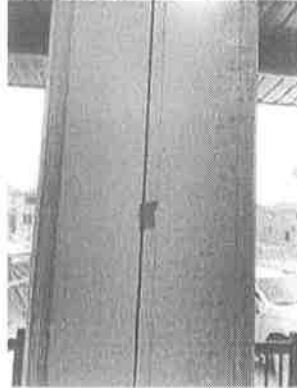
151397 - 1 - FRONT DOORS~CHIPS ON METAL ASTRAGAL AT FRONT DOORS
