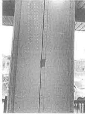
151397 - 1 - FRONT DOORS~CHIPS ON METAL ASTRAGAL AT FRONT DOORS
