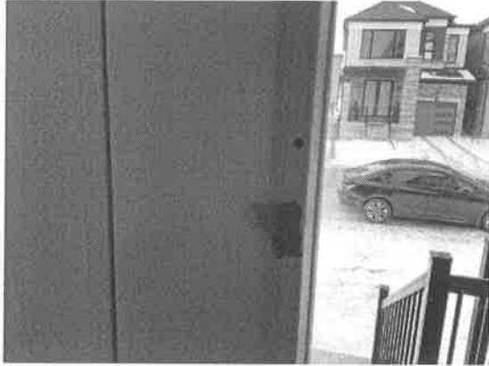
153414 - 1 - FRONT DOORS~SCREW CAP NOT INSTALLED AT RIGHT FIXED GLASS
