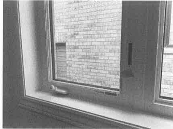
153400 - 1 - WINDOWS~WINDOW CRANK NOT INSTALLED
