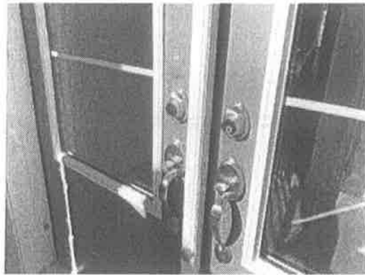
151939 - 1 - NOTE:~BLACK MARKS ON MIDDLE ASTRICAL AT FRONT DOOR
