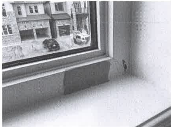
152122 - 1 - WINDOWS~CRACK ON RIGHT FIXED WINDOW MULLIN BOTTOM RIGHT CORNER
