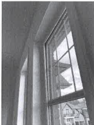
152121 - 1 - WINDOWS~ADJUST OPERATING WINDOW BOWED
