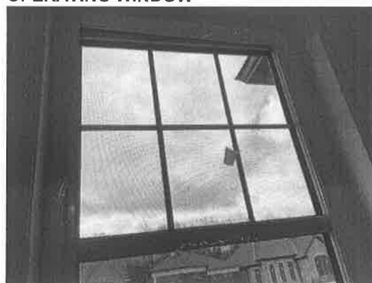
152142 - 1 - NOTE:~SCREEN RIPPED AT OPERATING WINDOW
