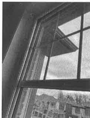
152143 - 1 - NOTE:~ADJUST WINDOW WILL NOT CLOSE
