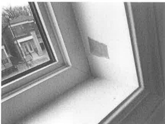
152130 - 1 - WINDOWS~CRACK ON RIGHT MULLIN RIGHT FIXED WINDOW
