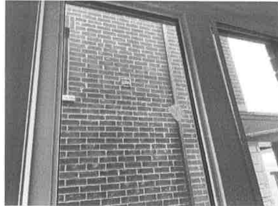
152566 - 1 - WINDOWS~SCRATCH ON LEFT FIXED GLASS LEFT OF OPERATING WINDOW AT DINNING FROM FOYER
