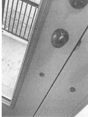
152563 - 1 - FRONT DOORS~MISSING SCREW COVER BELOW HANDLE AT OPERATING DOOR
