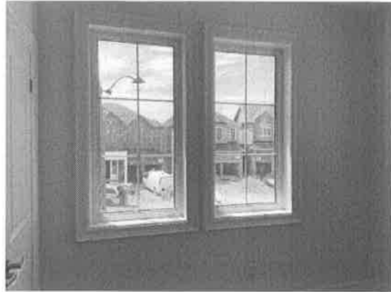
147653 - 2 - WINDOWS~CRACKED FIXED GLASS LEFT WINDOW
