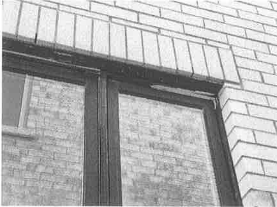
150365 - 2 - frame - Scratches on right fixed window at exterior and frame broken
