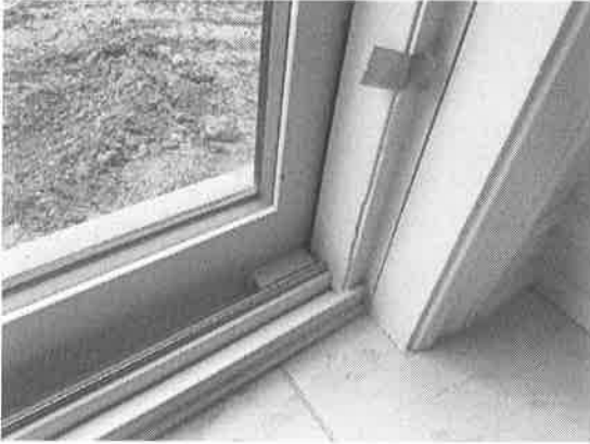
150267 - 1 - WINDOWS~DAMAGE WINDOW TRIM RIGHT SIDE
