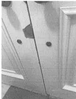
151197 - 1 - NOTE:~CHIPS ON ASTRAGAL AT FRONT DOOR.
