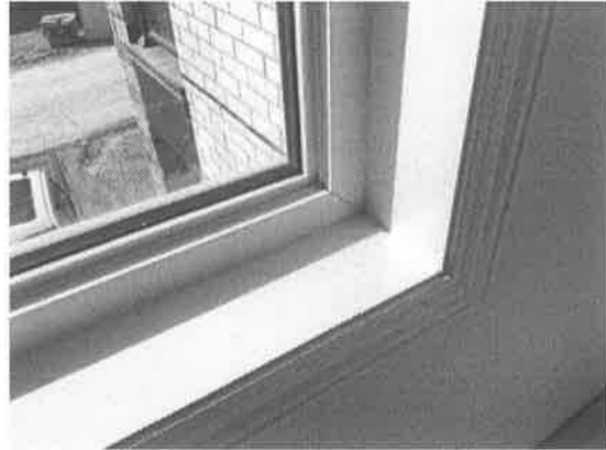
150998 - 2 - WINDOWS~CRACKED MULIN FROM INTERIOR
