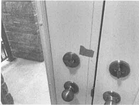
151102 - 1 - FRONT DOORS~CHIP ON ASTRAL AT FRONT DOOR
