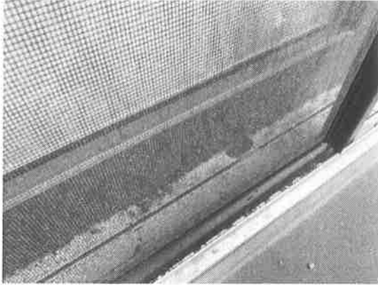
151096 - 1 - NOTE:~DAMAGE THRESHOLD AT REAR OF HOME AT BALCONY SLIDING DOOR LEFT SIDE
