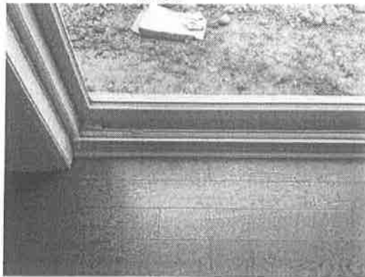
149289 - 1 - WINDOWS~DENT ON LEFT SLIDING DOOR TRIM AT BASE
