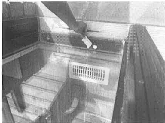
149109 - 1 - 1 - item 30- 2nd floor sliding black exterior mullin cracked on left side where door opens
