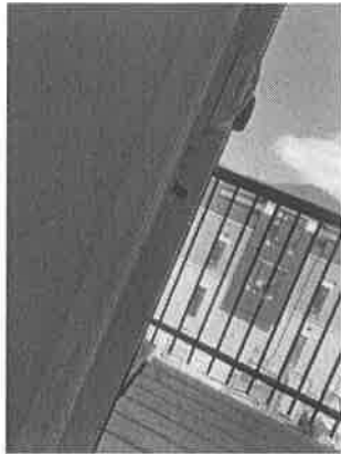
147350 - 1 - WINDOWS~LEFT MULLIN CRACKED AT BALCONY DOOR
