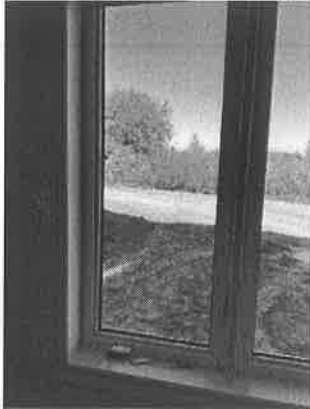
150532 - 2 - WINDOWS~SCREEN NOT INSTALLED AND INSIDE LIVING ROOM- INSPECT BOWED SCREEN THROUGHOUT NOT FITTING PROPERLY
