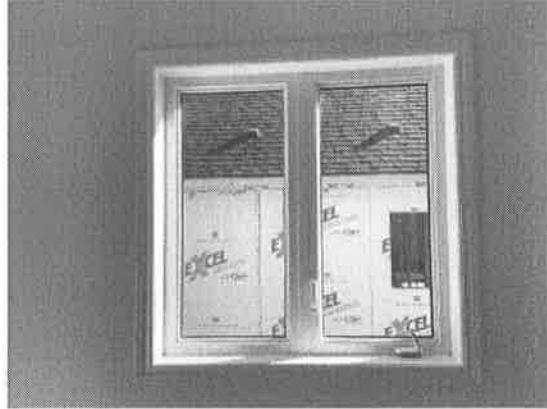
150532 - 1 - WINDOWS~SCREEN NOT INSTALLED AND INSIDE LIVING ROOM- INSPECT BOWED SCREEN THROUGHOUT NOT FITTING PROPERLY
