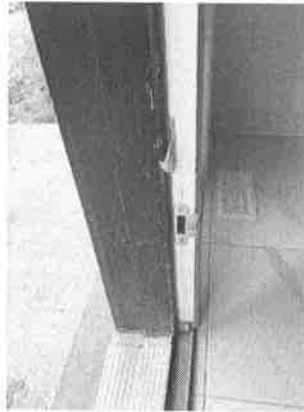
148722 - 1 - FRONT DOORS~CRACK INSIDE TRIM BELOW HINGES AT FRONT DOOR
