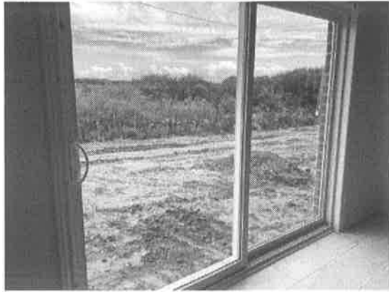
150050 - 1 - WINDOWS~SCREEN DOOR NOT INSTALLED AT SLIDING DOOR
