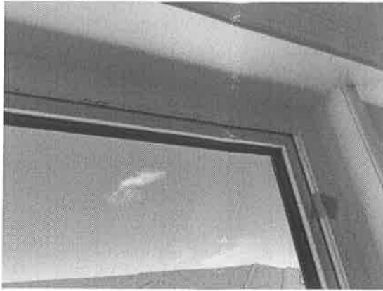
148397 - 1 - WINDOWS~DAMAGED WINDOW TRIM AT OPERATING WINDOW
