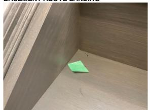
149356 - 3 - STAIRS~VARNISH REQUIRED AT TRIM RIGHT OF OUTSIDE STRINGER BY STAIRS TO BASEMENT / VARNISH DRIP MARK ON TREAD ABOVE LANDING TO BASEMENT STAIR / VARNISH CHIP ON TREAD AT STAIRS TO BASEMENT ABOVE LANDING
