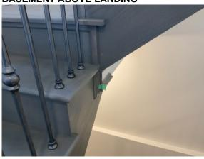
149356 - 2 - STAIRS~VARNISH REQUIRED AT TRIM RIGHT OF OUTSIDE STRINGER BY STAIRS TO BASEMENT / VARNISH DRIP MARK ON TREAD ABOVE LANDING TO BASEMENT STAIR / VARNISH CHIP ON TREAD AT STAIRS TO BASEMENT ABOVE LANDING
