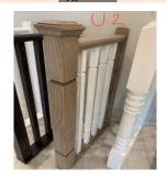
1 5/16" "V" Groove design in PAINT GRADE (Poplar) and PRE-FINISHED with a SEMI-GLOSS WHITE PAINT 3"  $\times$  1-3/4" Traditional handrail (with a steel bar insert) -- OAK 3 1/2"  $\times$  3 1/2" "V" Groove design with no Cap (Square cut) in OAK - as required
