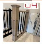
5/8" Round metal & cast iron picket alternating between No. LFOB-115TP and No. LFOB-115NC with both having No. E58 shoes and painted in a satin black colour 3" x 1-3/4" Centurion (profile # 15) handrail (with a steel bar insert) -- OAK 3-1/2" x 3-1/2" newel post P-590 with deocrative cap -- OAK
